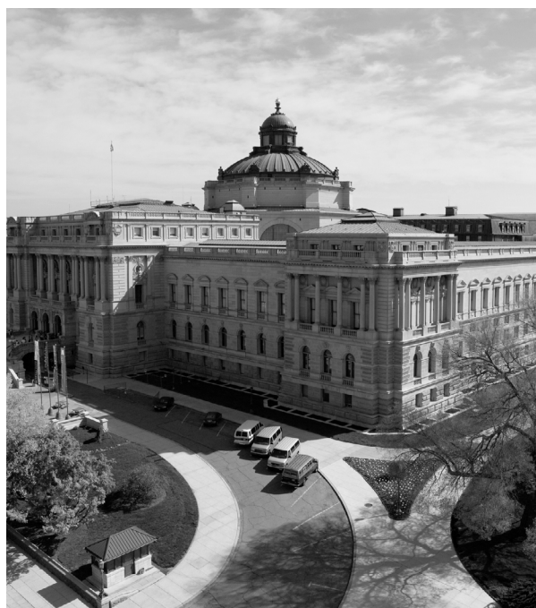
The Library's Jefferson Building
